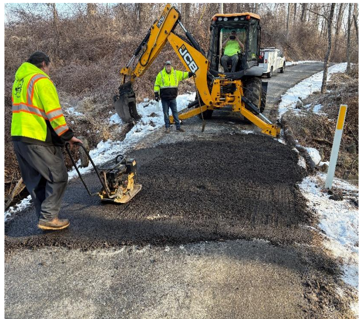
Yeatmans Station Culvert temporary repair
