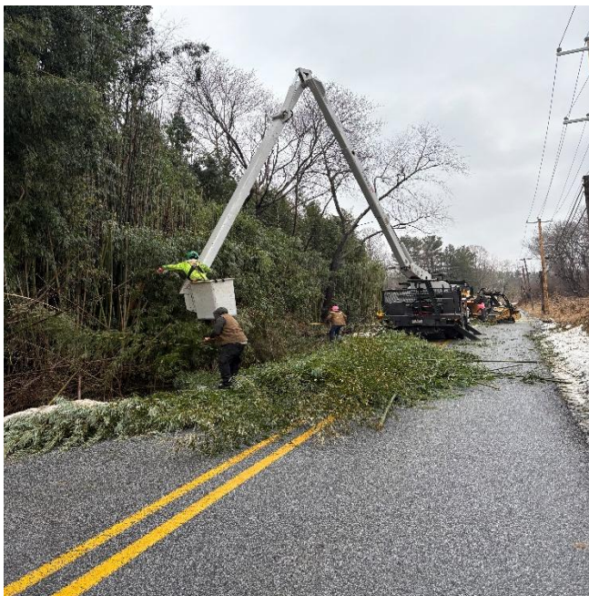
Chesterville Road Bamboo removal
