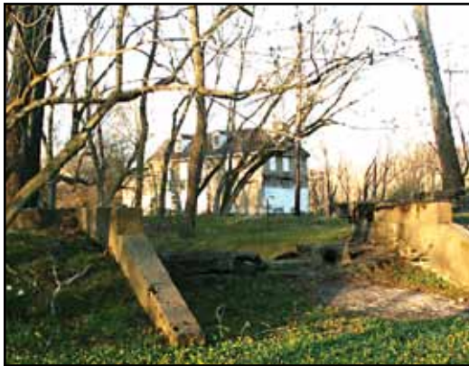
Across the street from the house is the original millrace, which at one time allowed the water of the mill pond to flow to the mill.
